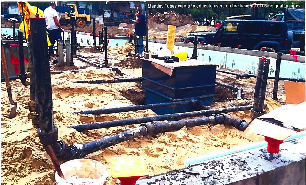
Installation of pipe couplings.
